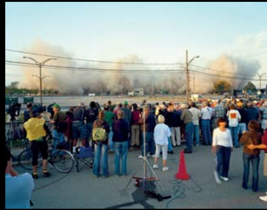
Demolition of Buildings #65 & #69, Kodak Park, Rochester (2007)
